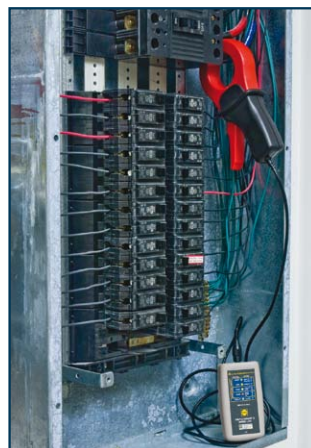
L101 recording branch circuit current.
